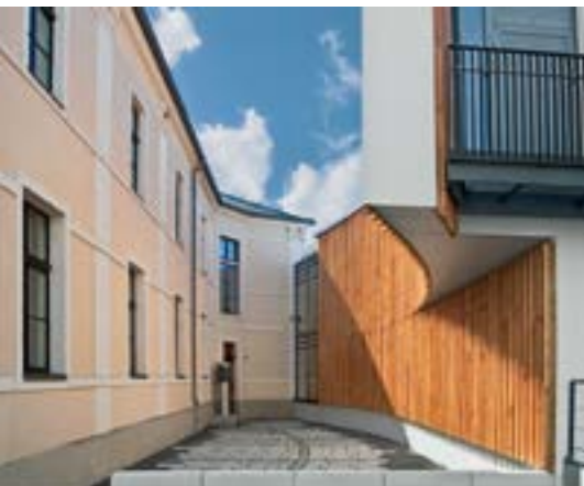
New storage building at the Völkerkundemuseum Herrnhut
